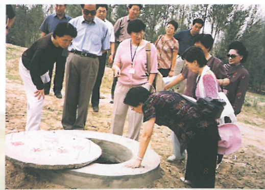
訪問團成員於八月五日往內蒙古涼城縣實地考察水窖的建造情況。 On 5 August 2001, our Delegation visited the Inner Mongolia to study the construction of wells.
